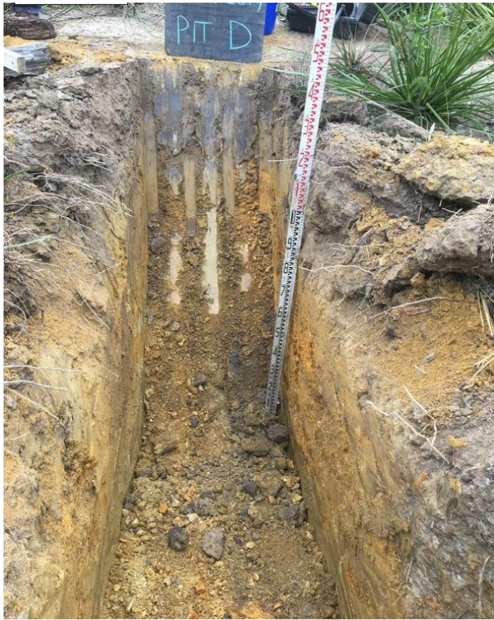
Figure 4. Test Pitting at NBR Project as part of Hydrogeology field studies
