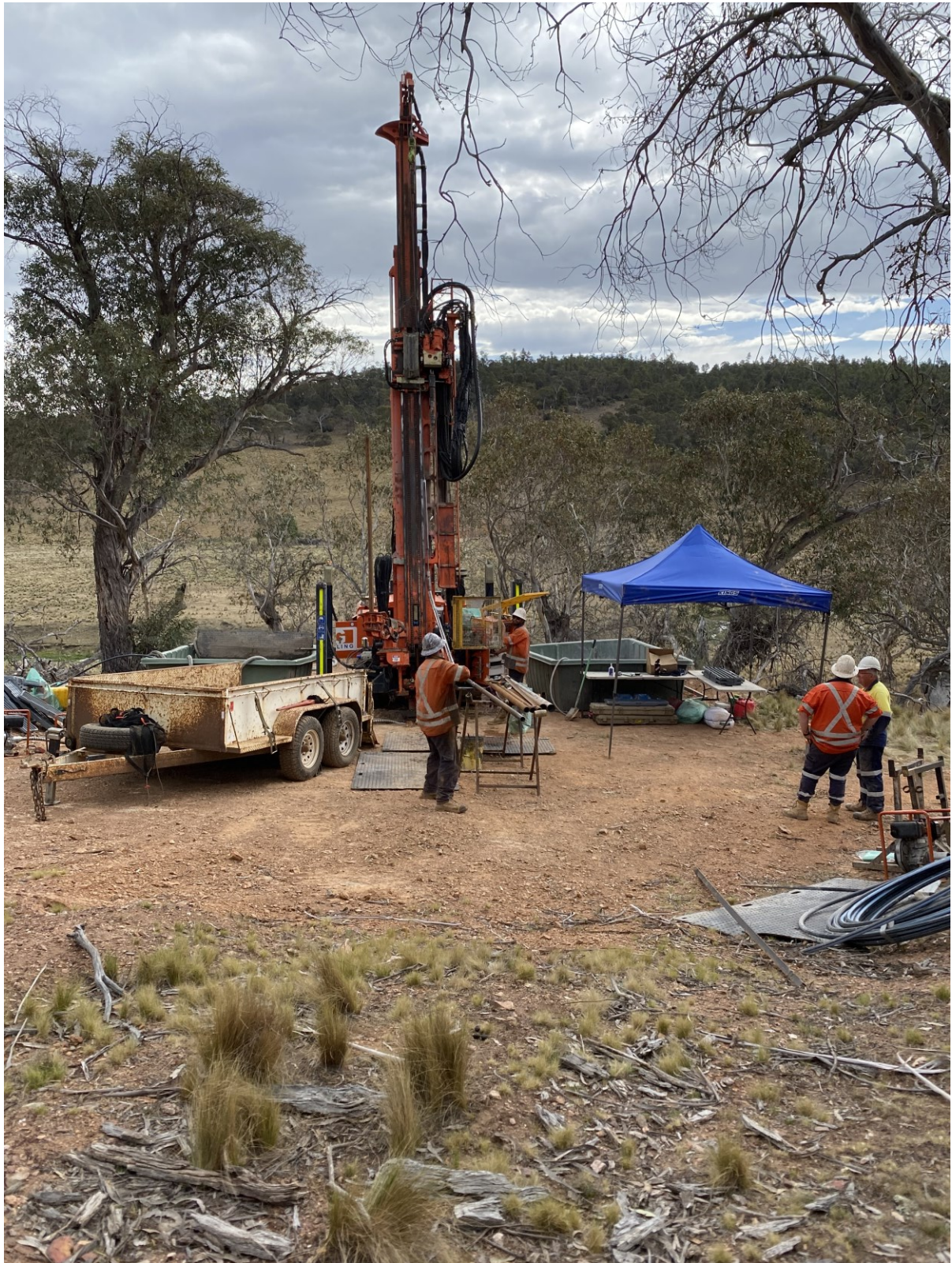
Figure 1: Drill Rig in operation at Rock Lodge
